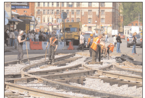
Below: Contemporary technology for rebuilding track. Good if they will be covered just with gravel and asphalt afterwards; in some cases they cover the wooden sleepers with concrete. The wood soon rots, and the road surface will be destroyed within two to three years after repair. V. Waldin
